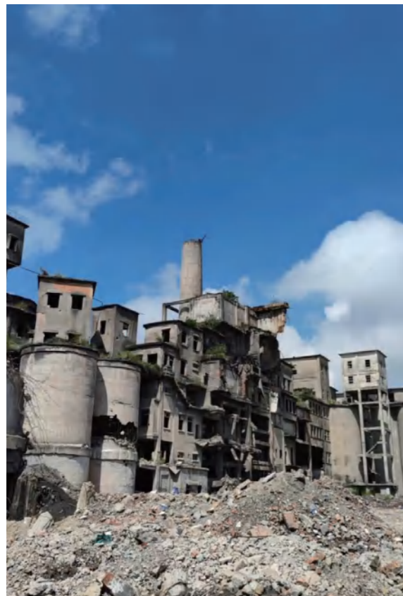
Cement Plant before renovation
