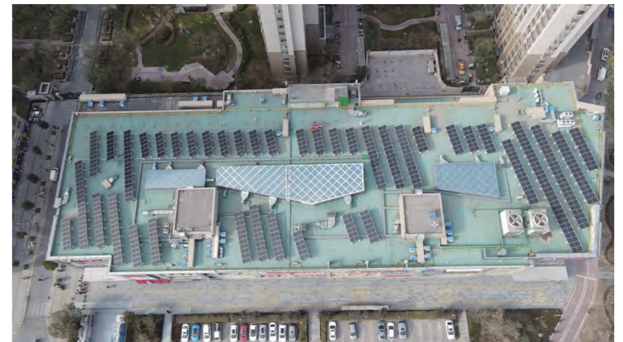
PV Application in Yinchuan Around the World
